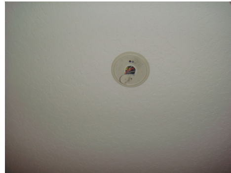
Missing smoke detector
